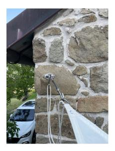
4. Attach first the sail "C" with the rope. Only in a second step shorten the distance using the hook.
